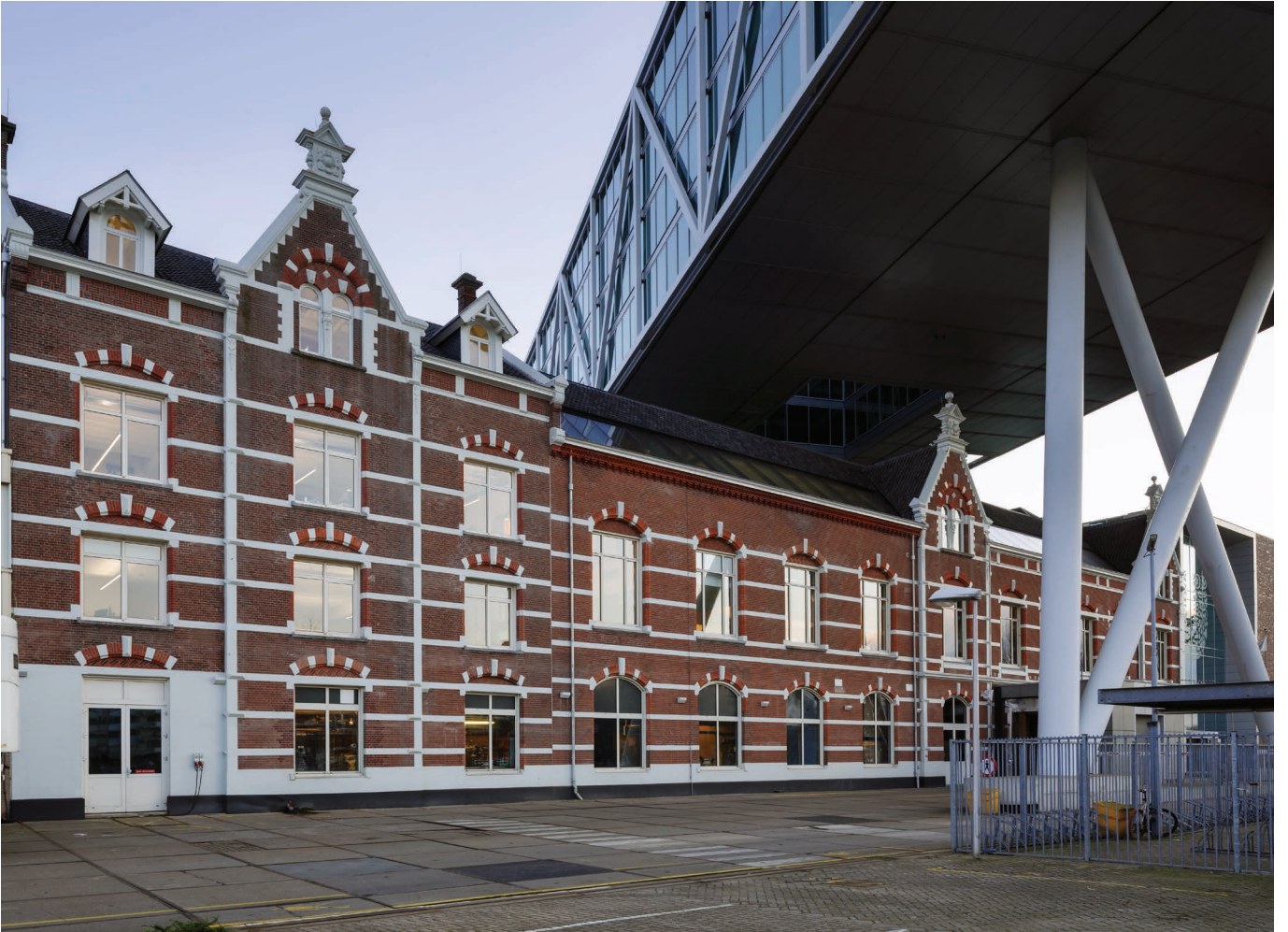
The tiled roof has been replaced by glass without impairing the original building.
