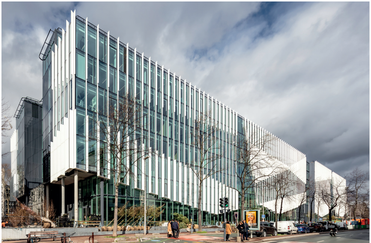
The façade, facing rue Colonel Pierre Avia, with its vertical fin shaders. (Paris 15th arrondissement)
