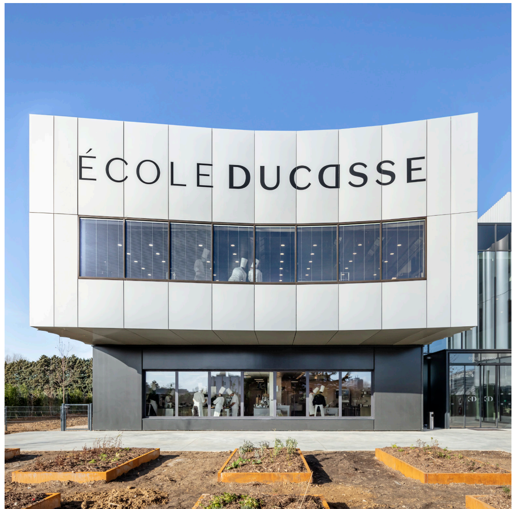
Concrete base, superstructure in glass and brushed metal.
