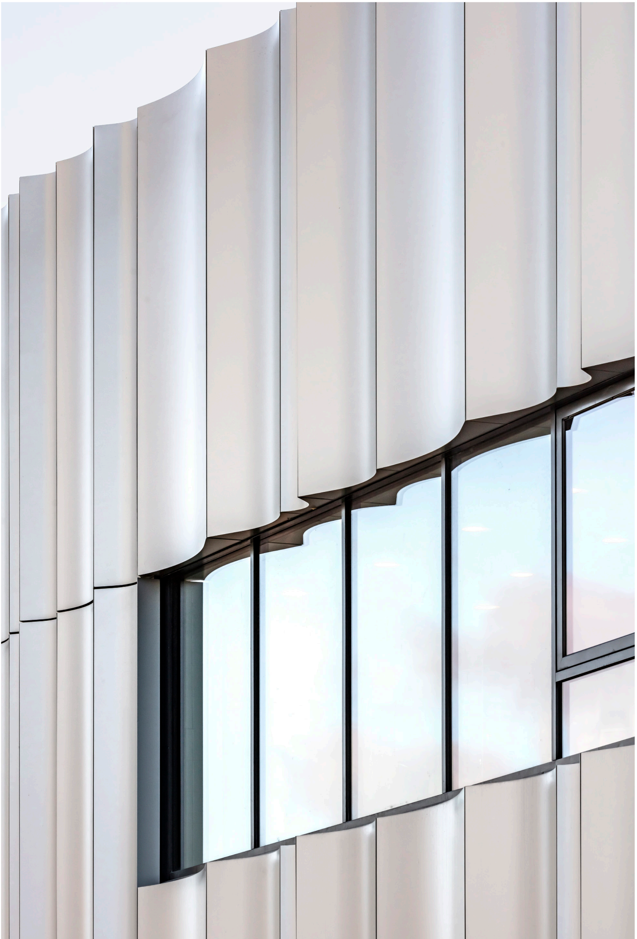
The undulating metal skin on the main body of the building
