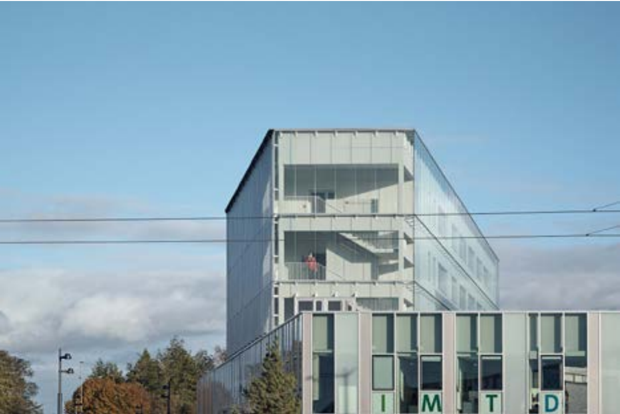
The double-skin principle of the facades allows users to take full advantage of solar gain while guaranteeing acoustic, solar protection in summer and thermal protection in winter.
