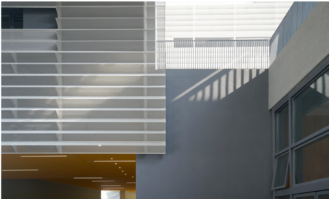
detail showing perforated panels
