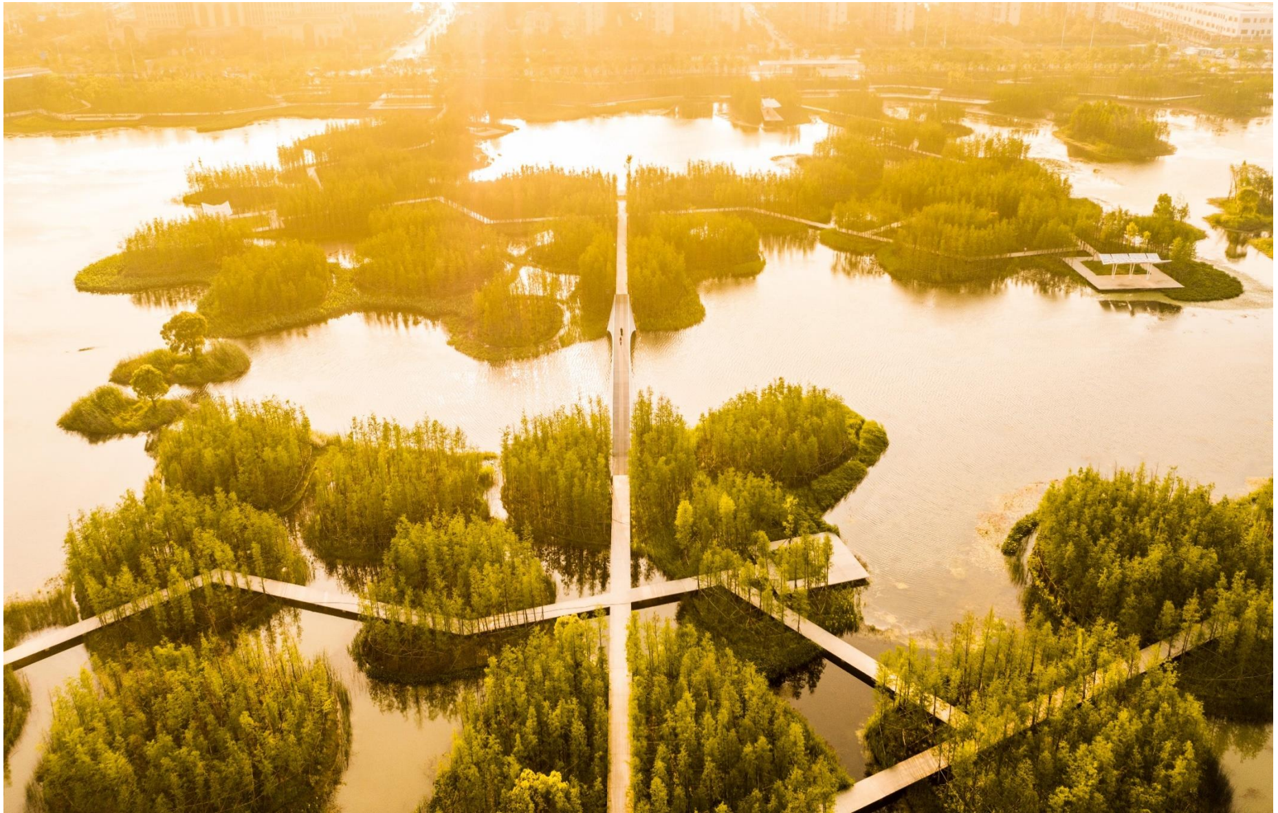
07. The lake with floating forest is able to accommodate two meters (6.5 feet) of water-level rise, providing the capacity to catch a full 1 million cubic meters of storm water inflow.
