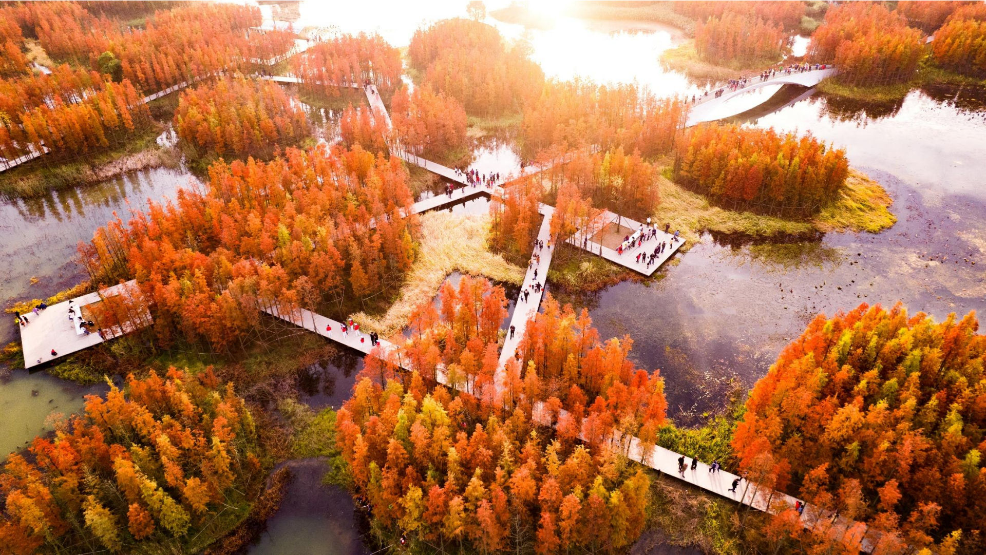
6. A network of boardwalk and platforms offers visitors an immersive contact with nature, which can be submerged during 20-year flood events and annual monsoon floods, which render the central part of the park inaccessible for several days. 6
