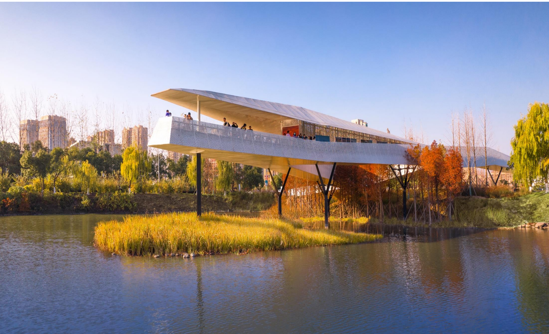
15 At the main entrance, an overpass is integrated with an art gallery and cafeteria, providing a day and night attraction. At the end of the overpass is a pavilion overlooking Aixi Lake offering a sweeping vantage of the city's skyline
