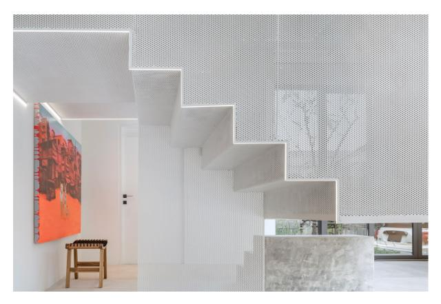
Since the stair is semi-transparent, it does not feel close-in or make the users uncomfortable to walk into. The steel sheets are well curated and geometrically folded to make thin steel sheets even stronger. So, the
