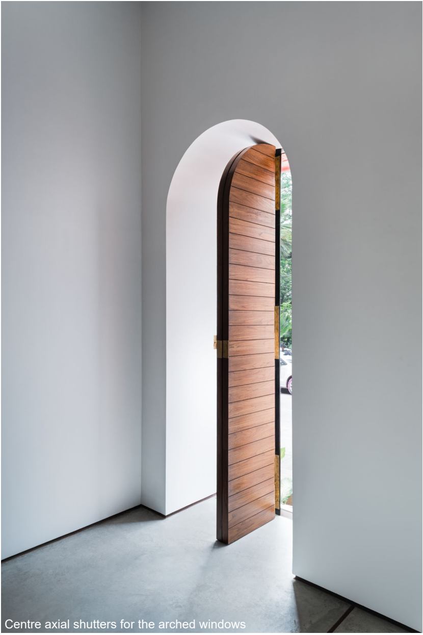
Centre axial shutters for the arched windows
