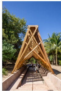
04 Orchid Pavilion_CCA_Foto Rafael Gamo. JPG & TIFF Image Description: Photography Image Credit: ©Photography Rafel Gamo courtesy of CCA Centro de Colaboración Arquitectónica
