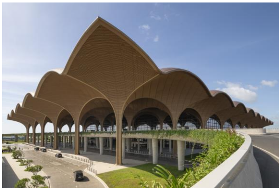
Techo International Airport by Foster + Partners Phnom Penh, Cambodia Jury Winner, Transportation Infrastructure Photo courtesy of Foster + Partners
