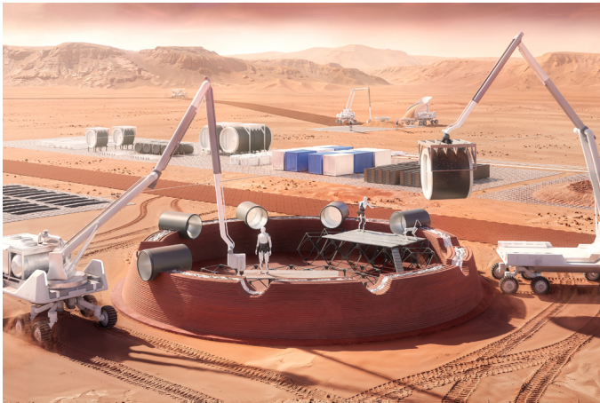
3D-printed construction of the habitat
