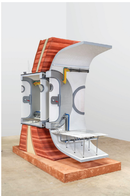
Sectional view of the wall assembly
