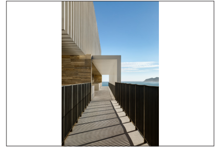
2018_SOLAZ_LOS_CABOS_SMA_PHOTO_by_ Rafael_Gamo_36.jpg Image Description: Exterior View - Circulations Image Credit: © Sordo Madaleno Arquitectos, photo by Rafael Gamo
