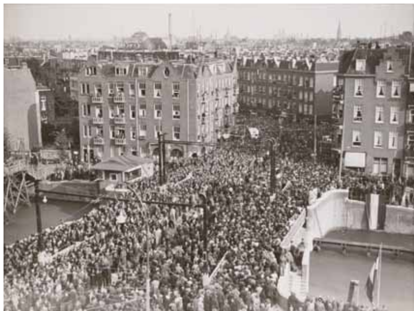
Massale belangstelling tijdens de opening van de Kinkerbrug (1937) Massive interest during the opening of Kinkerbrug (1937)
