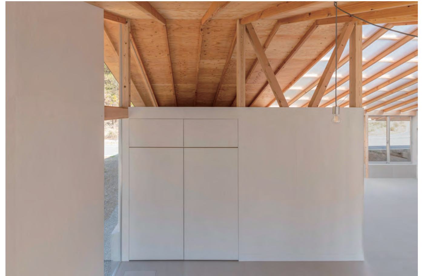
View loft from guest room. A conventional construction method using general metal fittings is used, and a bearing wall is installed in the center of the span to achieve a well-balanced arrangement. By using a cross, the line of sight is not obstructed and the space is a unified space.
