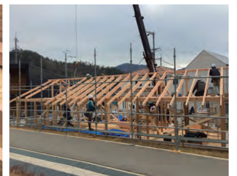
Wooden frame construction method.
