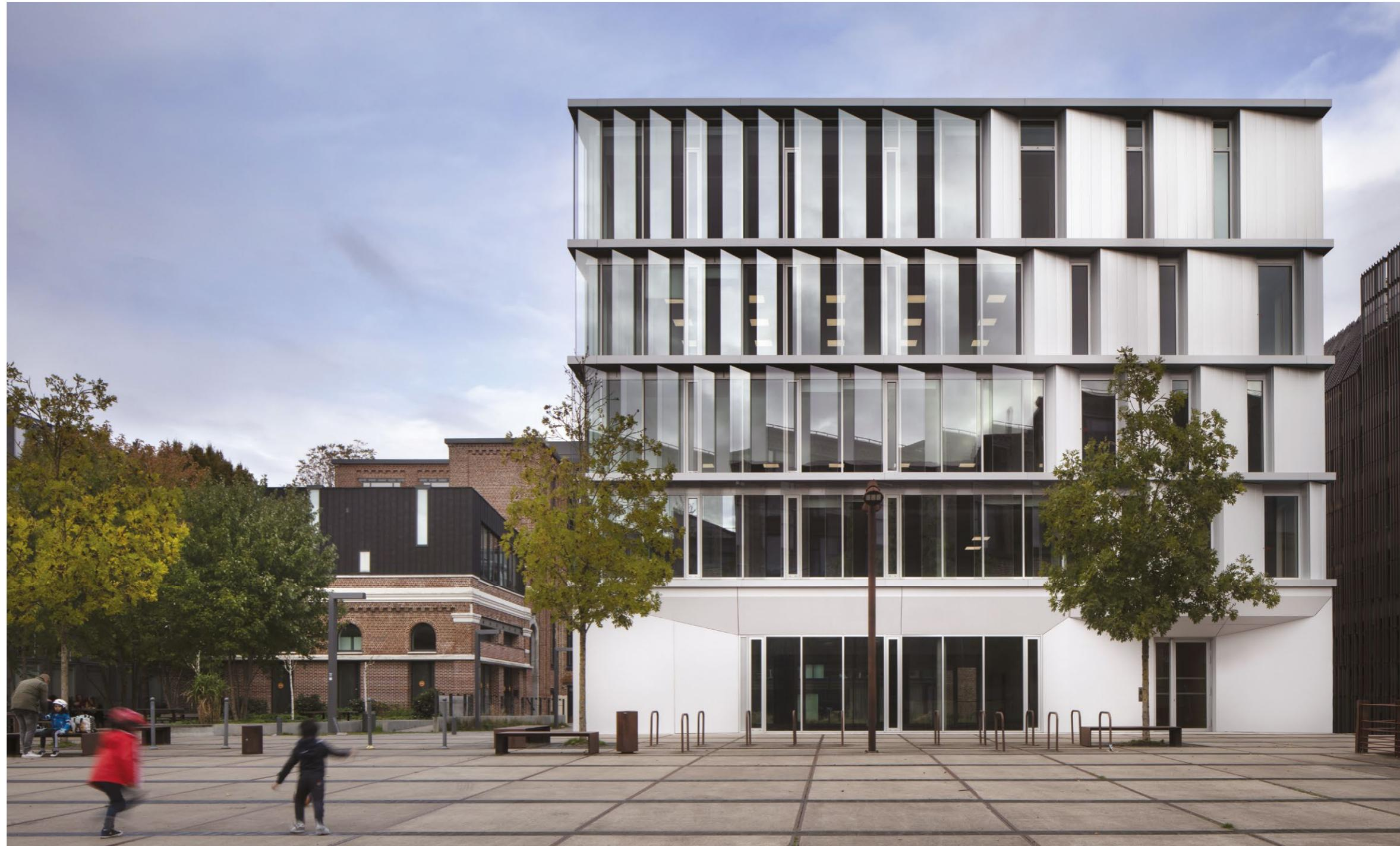
The vertical orientation of the glass louvers is chosen to protect from the southern sunrays and provide large visual perspectives. For the main facades - southwest and northwest - the project outlines the idea of a double skin that naturally creates a transparent and luminous curtain wall while protecting from the sunrays.
