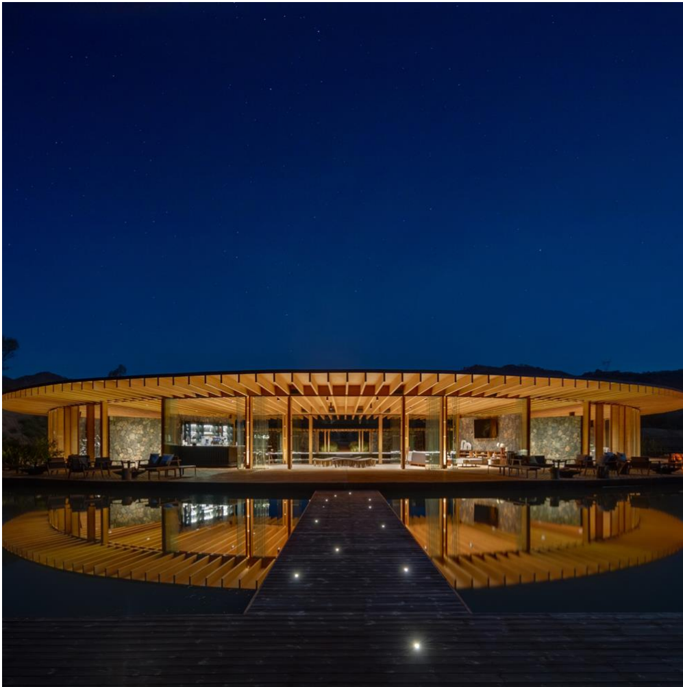
Above: Valle San Nicolás Clubhouse, Valle de Bravo, Mexico, by Sordo Madaleno Arquitectos
