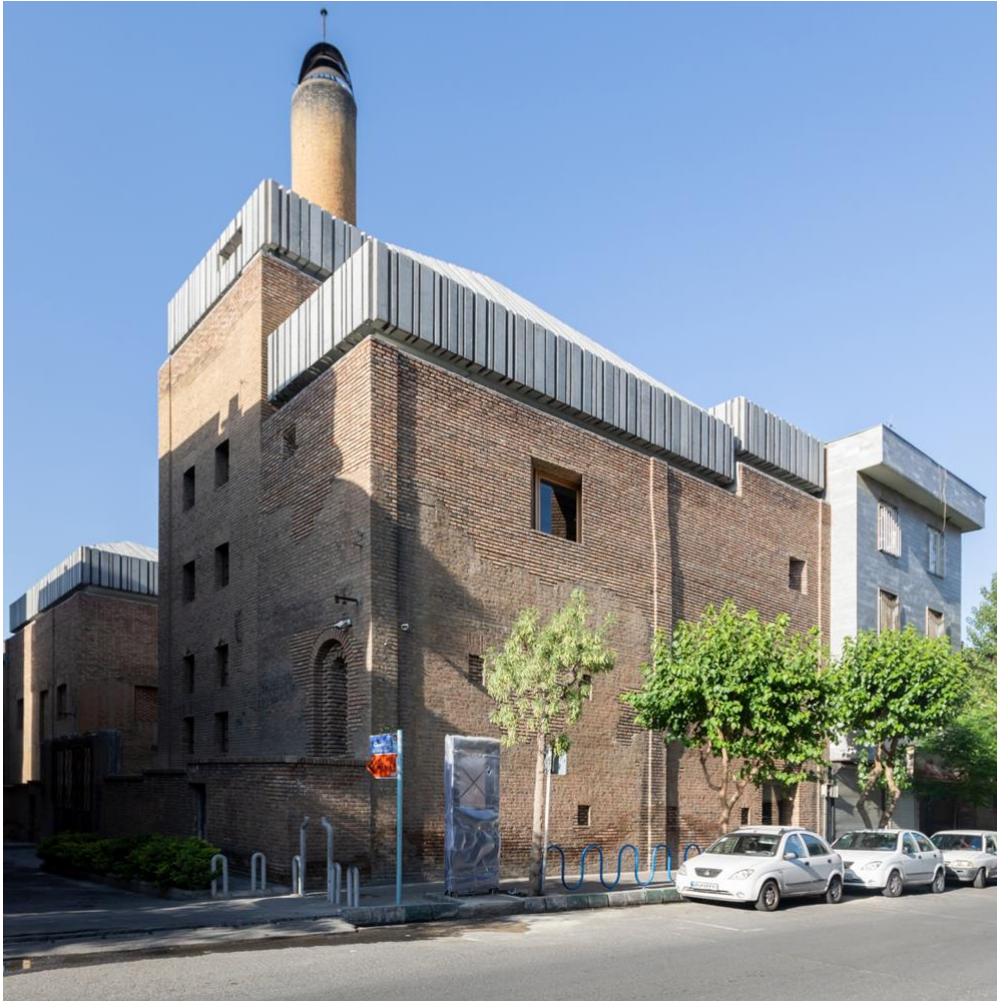
Above: Argo Contemporary Art Museum & Cultural Centre, Tehran, Iran, by Ahmadreza Schricker Architecture North. Image courtesy of Ahmadreza Schricker Architecture North
