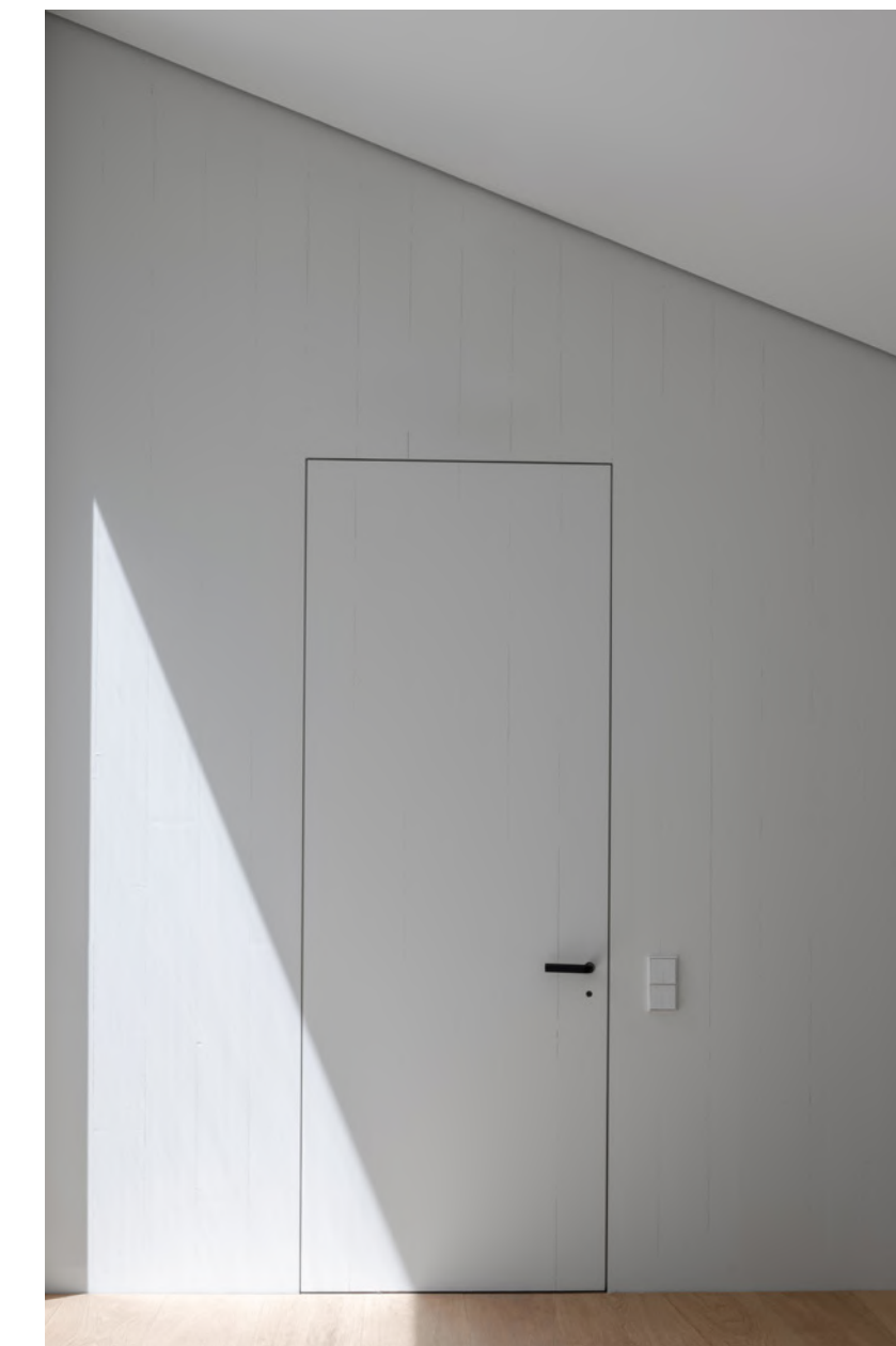
Hand crafted doors made out of the wall's masstimmer material let the wooden structure go through with only a minimal gap between.
