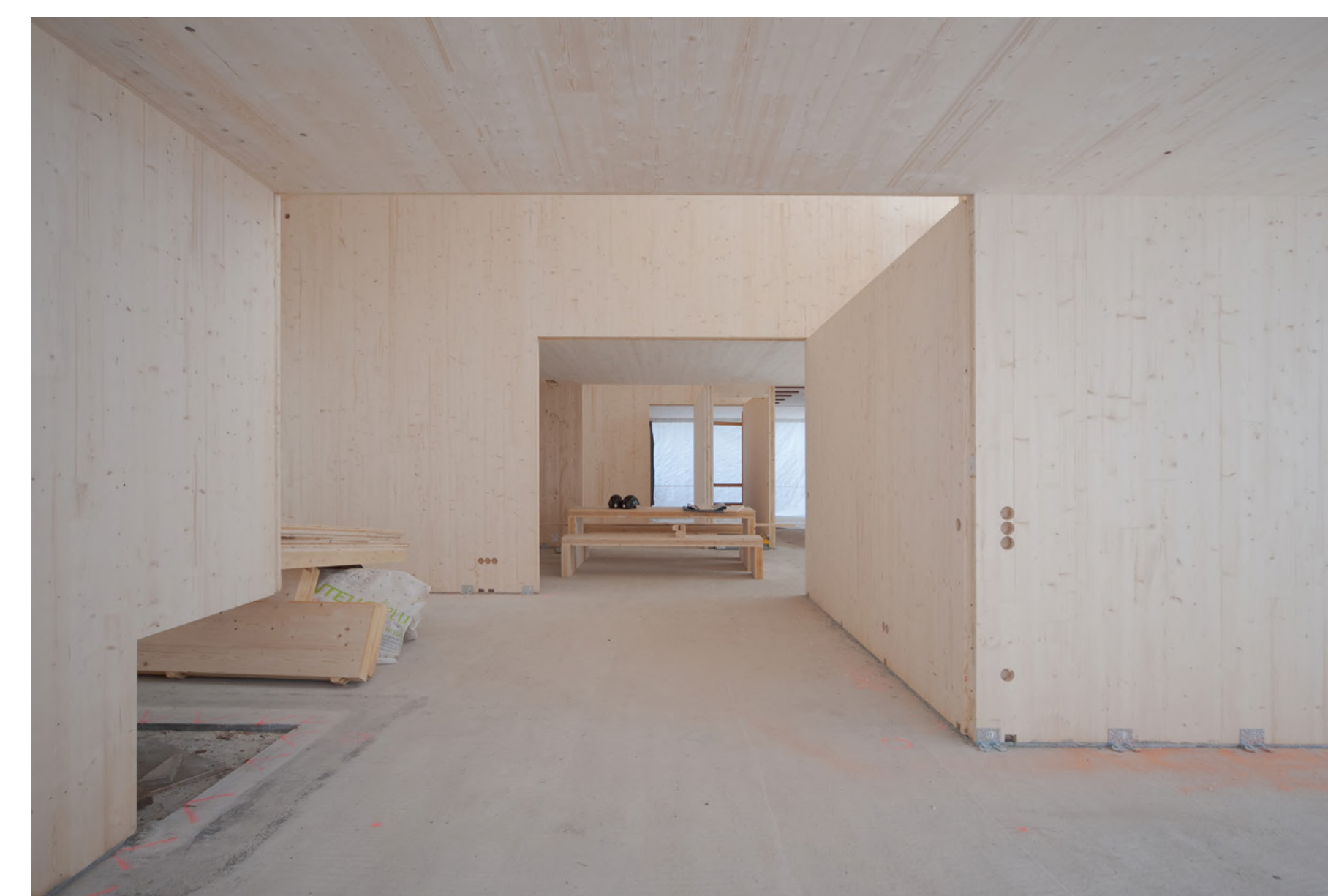
The mass timber during construction showing the cutout for the fireplace on the left.
