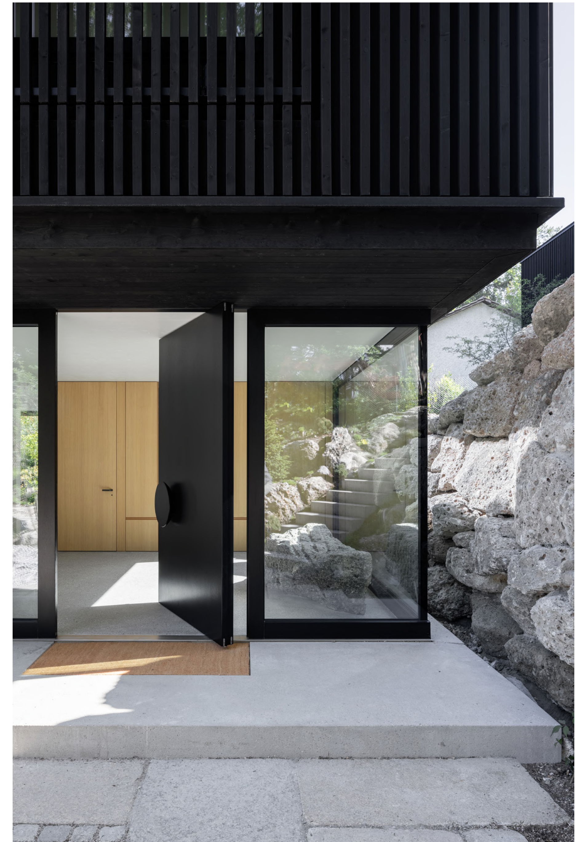
The covered entry outside and the entrance space with a rock embedded in the floor. The glas facade is not load bearing and the huge overhang of the box above is entirely held by a steel inforced timber construction by bringing this overhang in balance with the even bigger overhang above the living room on the other end of the building.
