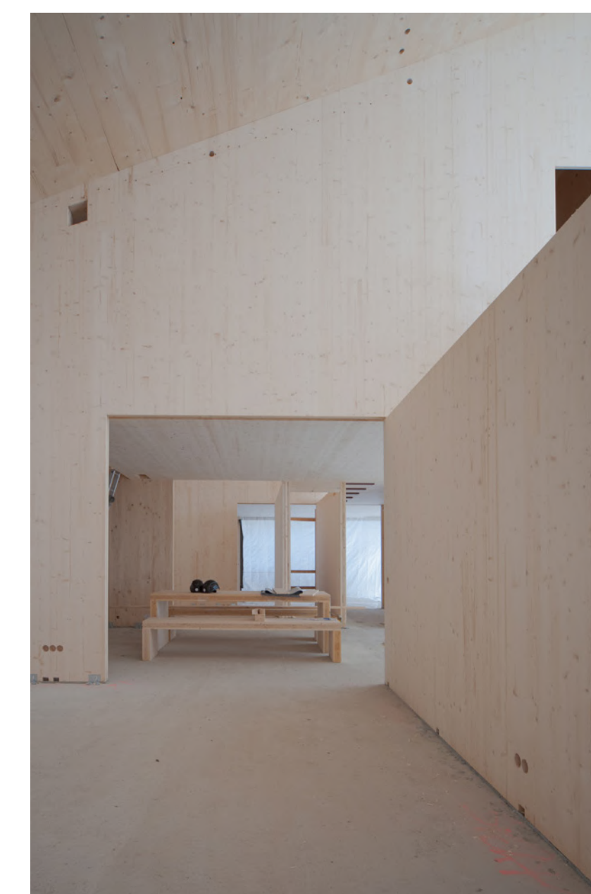
The mass timber during construction.
