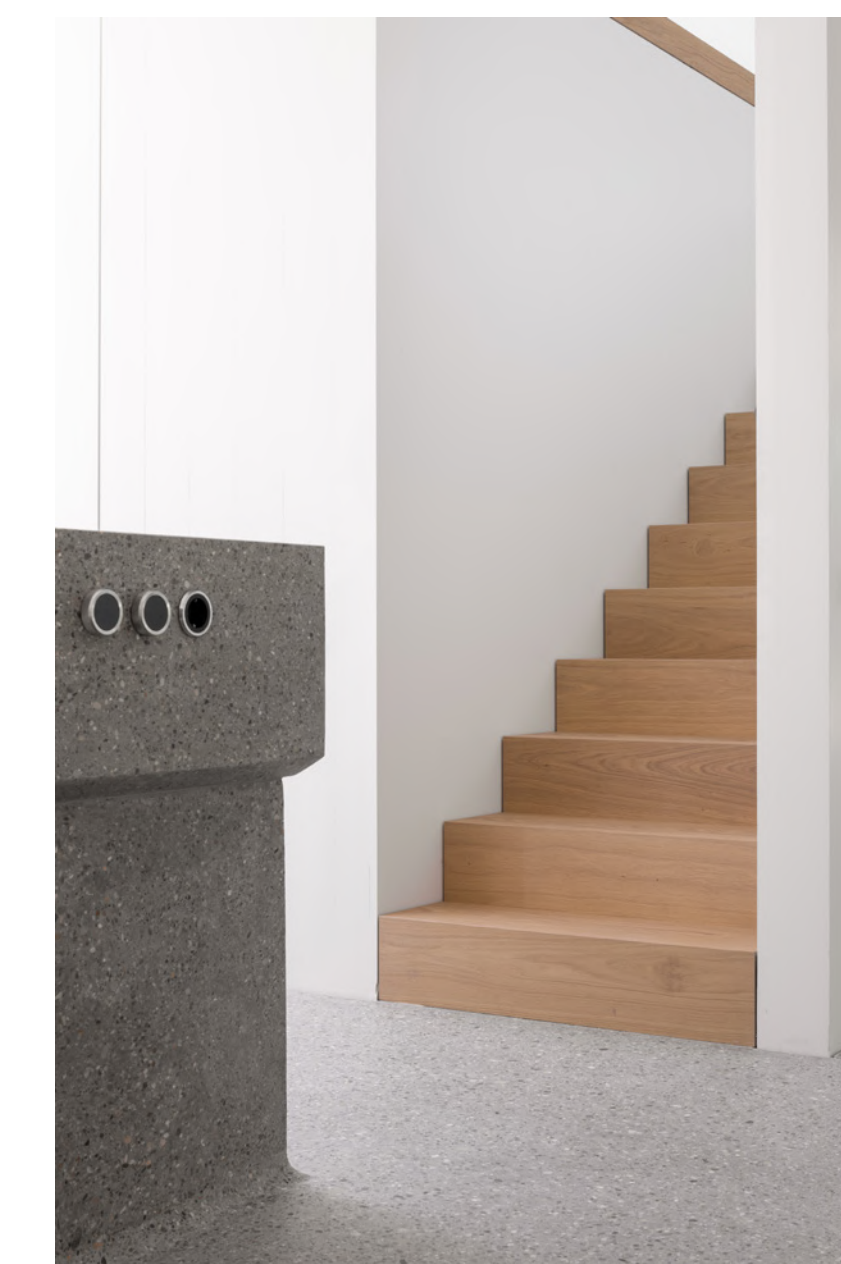
Detail of the kitchen block made in one piece jointless with the entire Terrazzo flooring.
