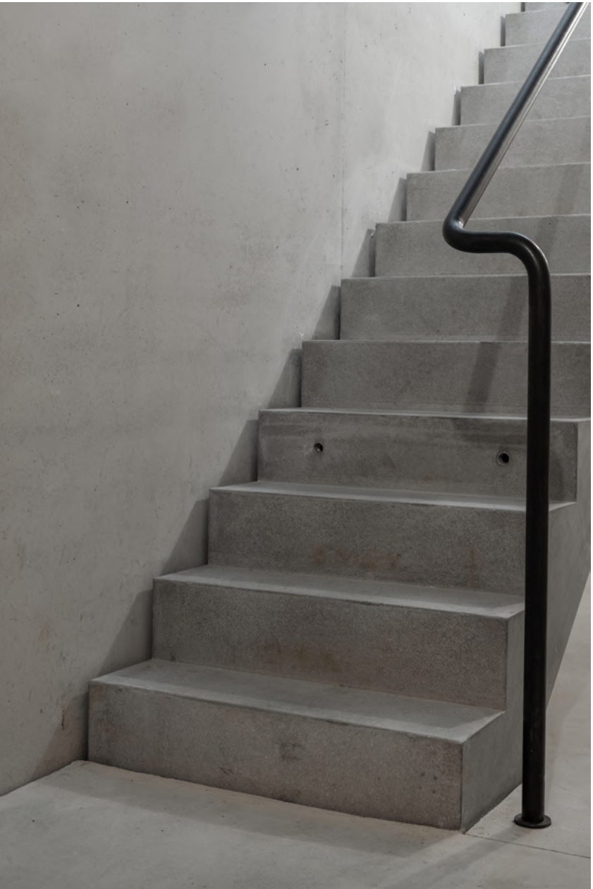
Detail of the steel handrail having only two fixingpoints.
