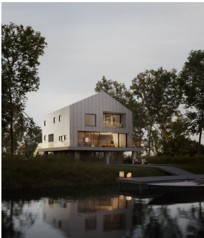
Tamsen House_FFA_02 © BS ARQ
