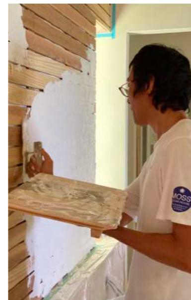
Plaster made from a mix of charcoal and effective microorganism (EM) bacteria provides a healthy, comfortable space by preventing mold and other putrefactive bacteria.
