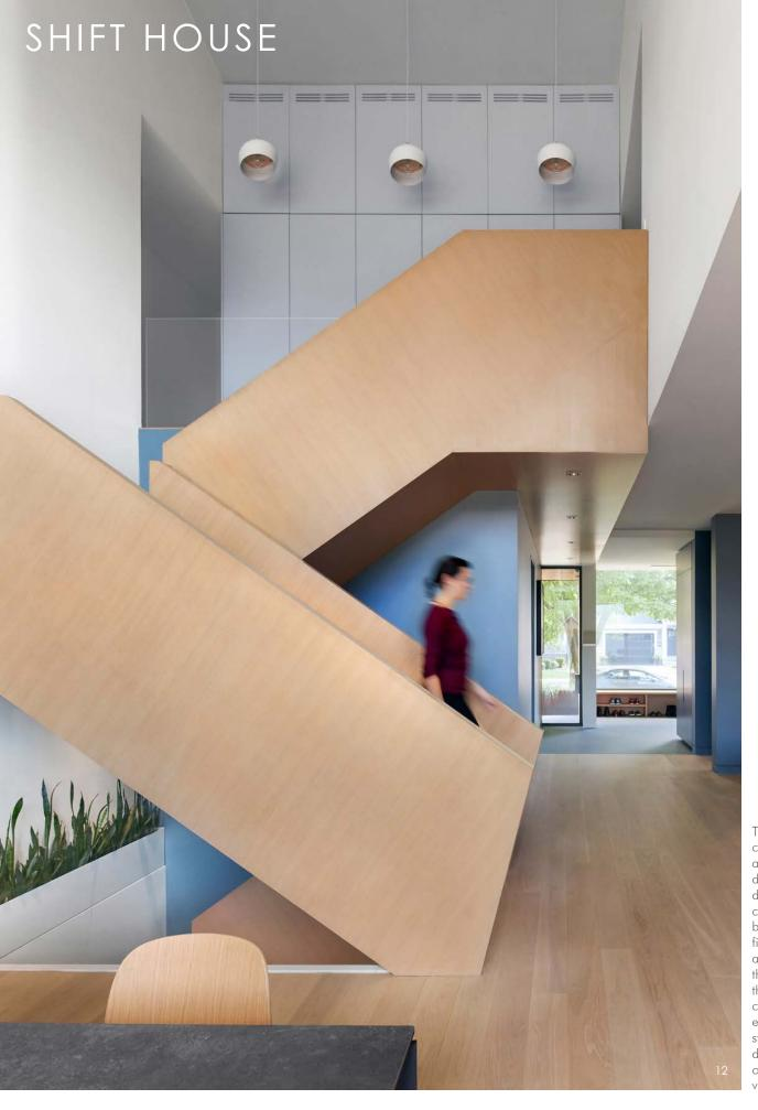
The stair's scissor configuration forms a compelling and dynamic threedimensional geometric composition, animated by the procession of figures as they ascend and descend between the different levels of the house. A woodclad ceiling treatment extends from the staircase to the foyer, defining the edge of one of the internal volumes.
