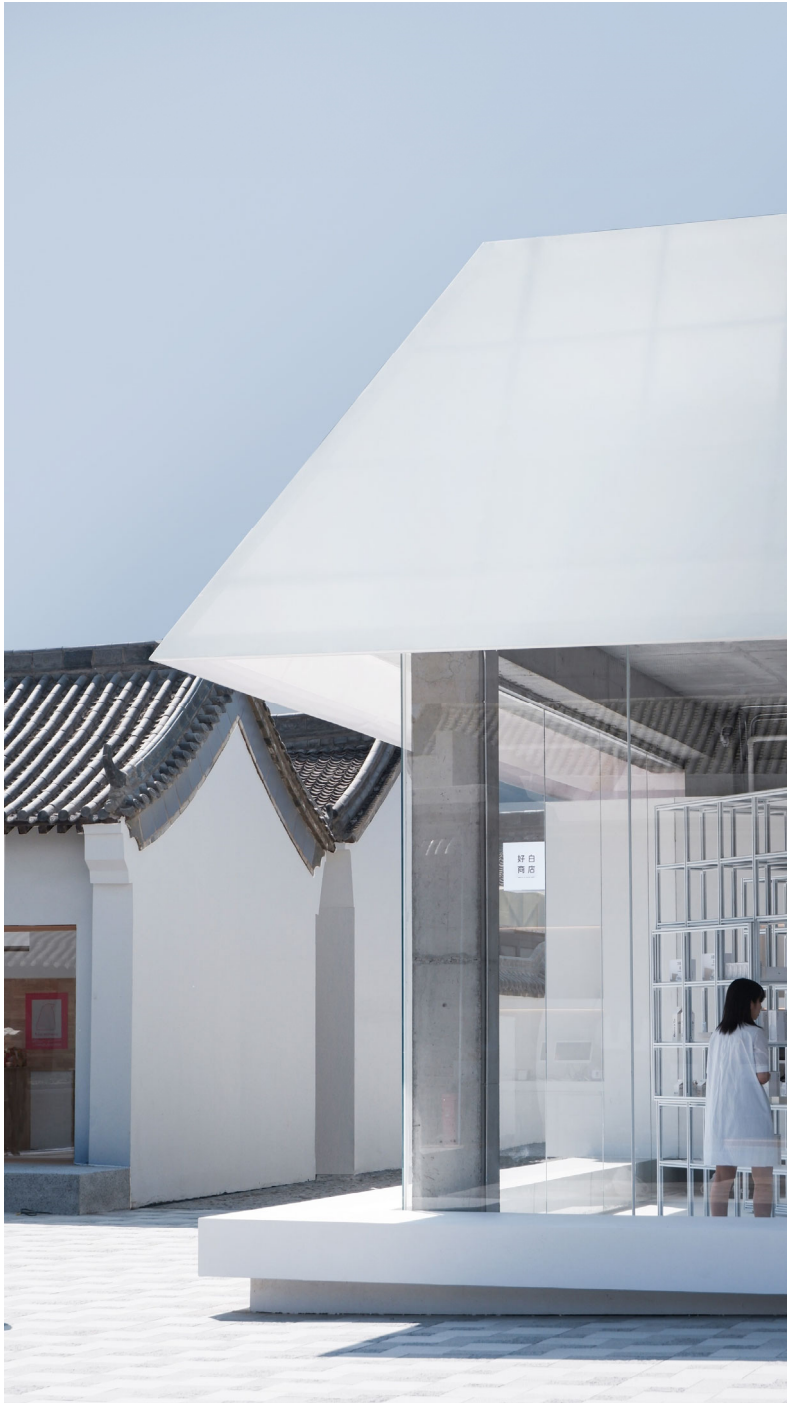
Close-up view towards corner of White Is Good Shop/ 好白商店转角立面的近景
