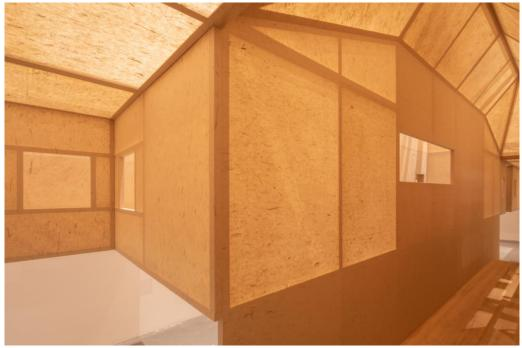
We chose handmade leatherette paper produced in Jing County, Anhui Province as the material for the spatial interface. This kind of paper has very clear fibers, thick and soft, transmits light appropriately, and gives people a warm feeling. The paper is lightweight, easy to hang, and can be replaced and maintained according to the needs of the exhibition.
