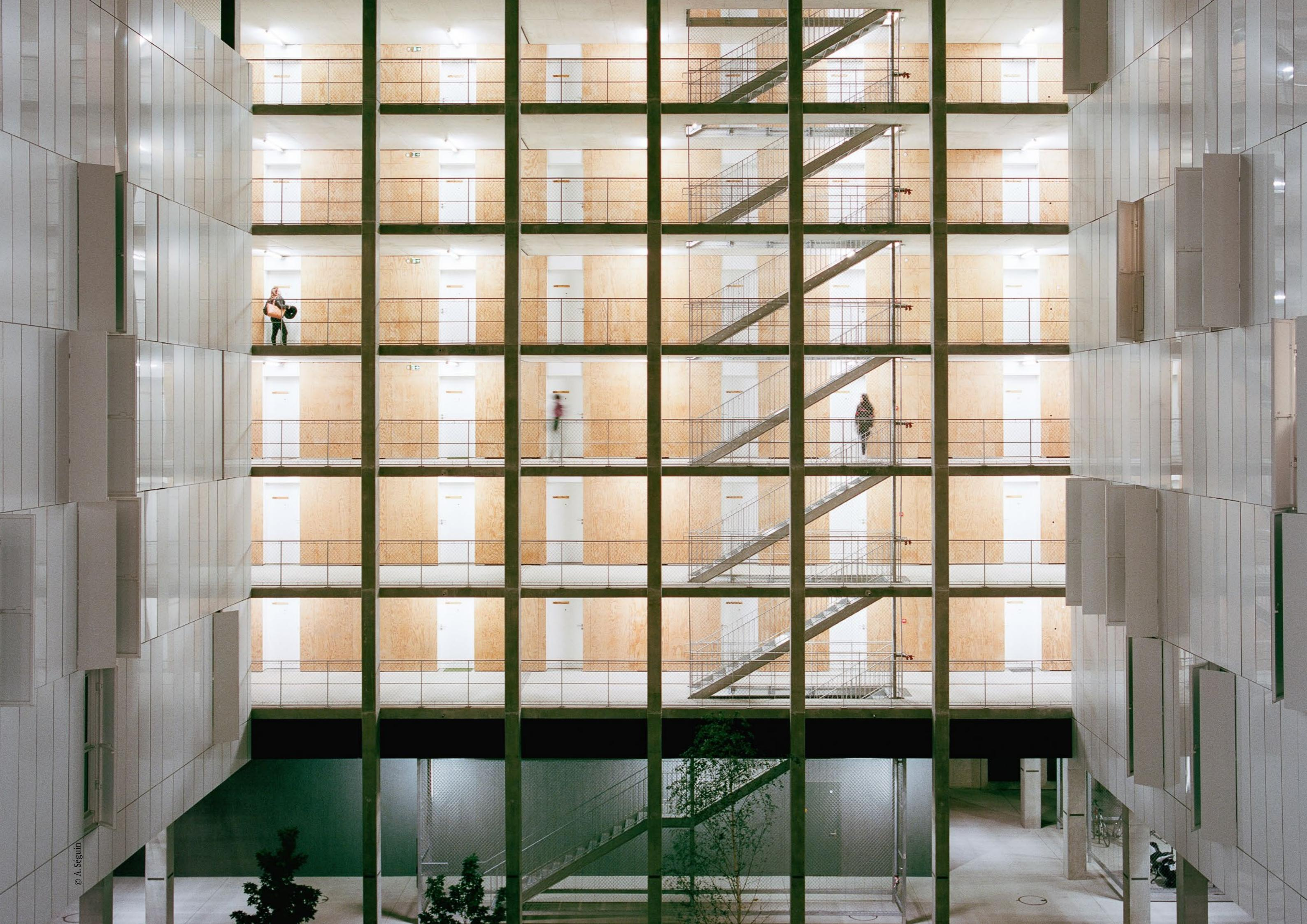
To the ancient, cloister-like arrangement of the volumes, replies the abstraction of the panels, which serve both as shutters and as cladding to the facade. Their dimensions rhythm the entire project, changing the perception of scale and diluting the beehive effect that might otherwise arise in the repetitive stacking of 615 lodgings. Always changing, this outer skin reacts as much to the reflections of its surroundings, as to the habits of its occupants.
